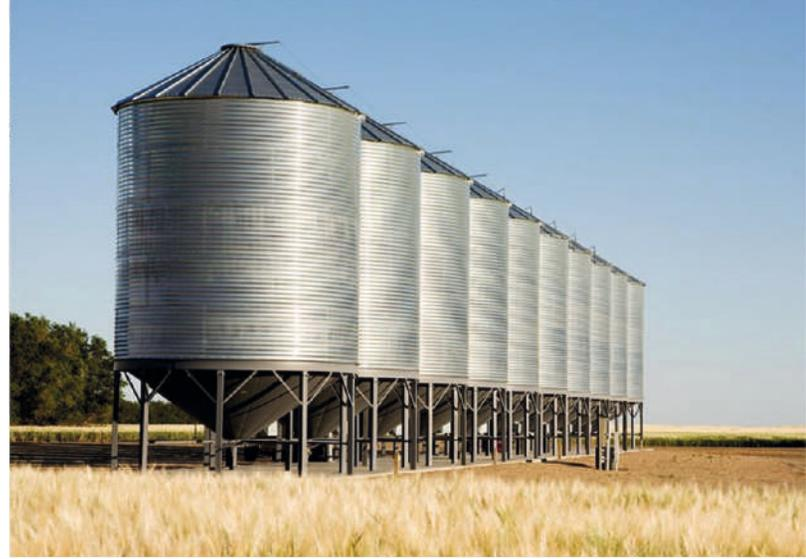
**Conical Bottom Silos;** are designed for short-term storage.
